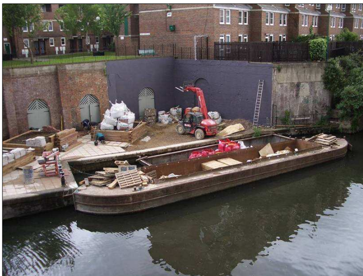
Photograph: Building materials being delivered to site by barge
